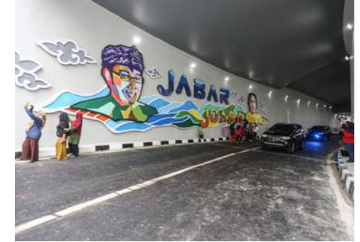
Underpass Depok – Nindya Karya
