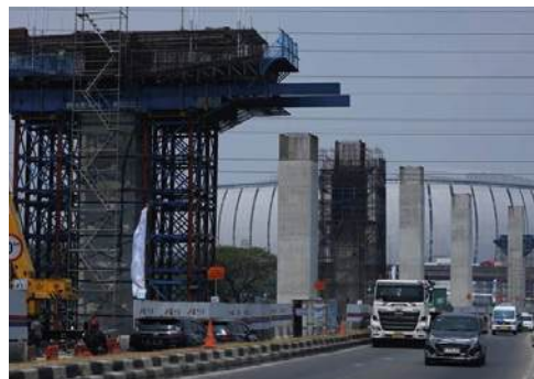
Jalan Tol Harbour Road II
