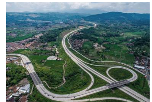
Jalan Tol Cisumdawu Seksi 5B – PT Girder
